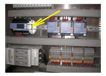
Fig 43: Example of physical size of remote PQ monitoring system
