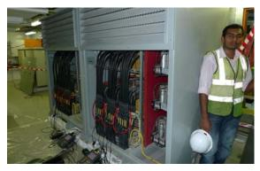
Fig 15: 2 x 2300HP/1800kW D type wide spectrum filters on mud pumps during ABS compliance testing in the UAE
