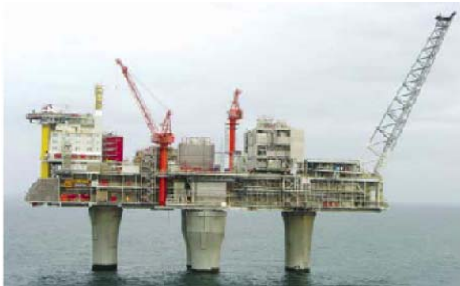
Fig 42 – The Norwegian Troll A gas platform. The 40MW HVDC enclosure is in the centre
