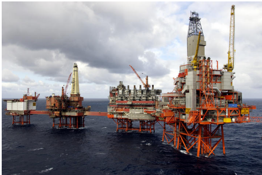
Fig 43 – BP Norway Valhall platform complex
