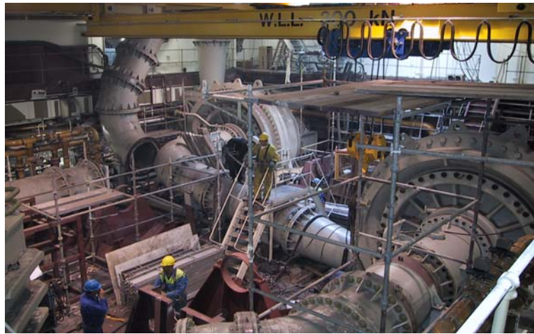
Fig 20 – Installation of 2 off 6MW dredge pumps, both VFD controlled (Bakker-Sliedrecht)
